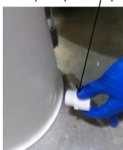
Thread the Cut Off pipe nipple into the new Male Pipe Adapter inside the chlorinator.
