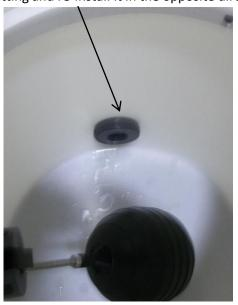
Thread the Cut Off pipe nipple into Bulk Head Fitting inside the chlorinator.
